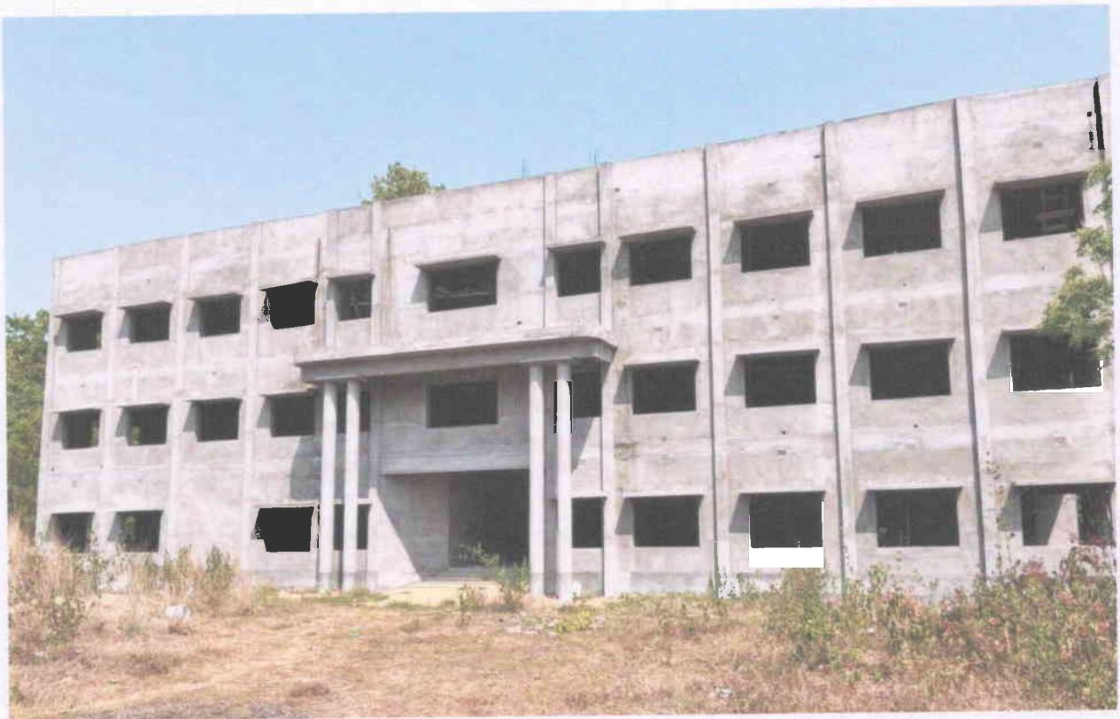
PG BUILDING (Under Construction)
